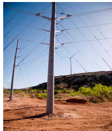
Figure 26. Composite Distribution Pole
