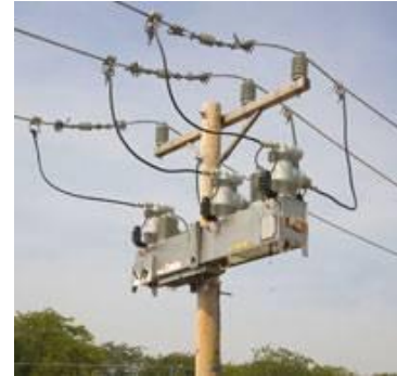
Figure 29. Installed IntelliRupter Recloser
