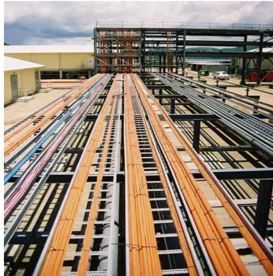
Figure 7. Cable Tray in a Refinery
