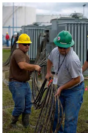
Figure 12. Portable Generator Cabling
