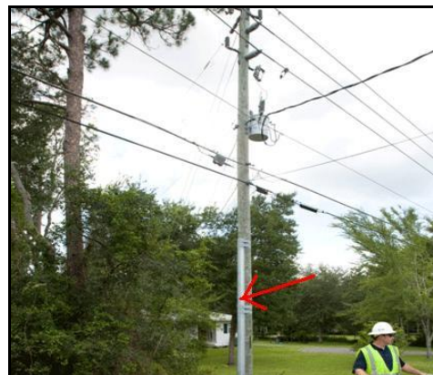
Figure 28. Osmose ET-Truss
