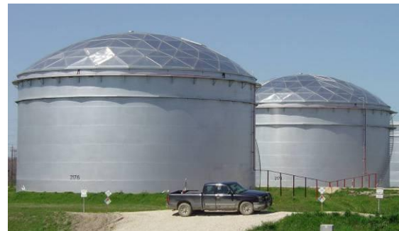
Figure 6. Wind Girders on Tanks
