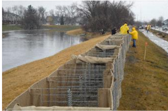
Figure 24. HESCO Floodline Concertainer Installation
