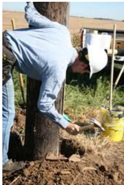
Figure 21. Wood Pole Being Sounded
