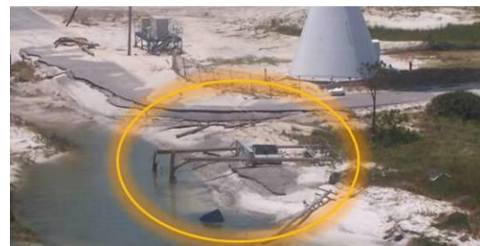
Figure 18. Underwater Cable Crossing Exposed
